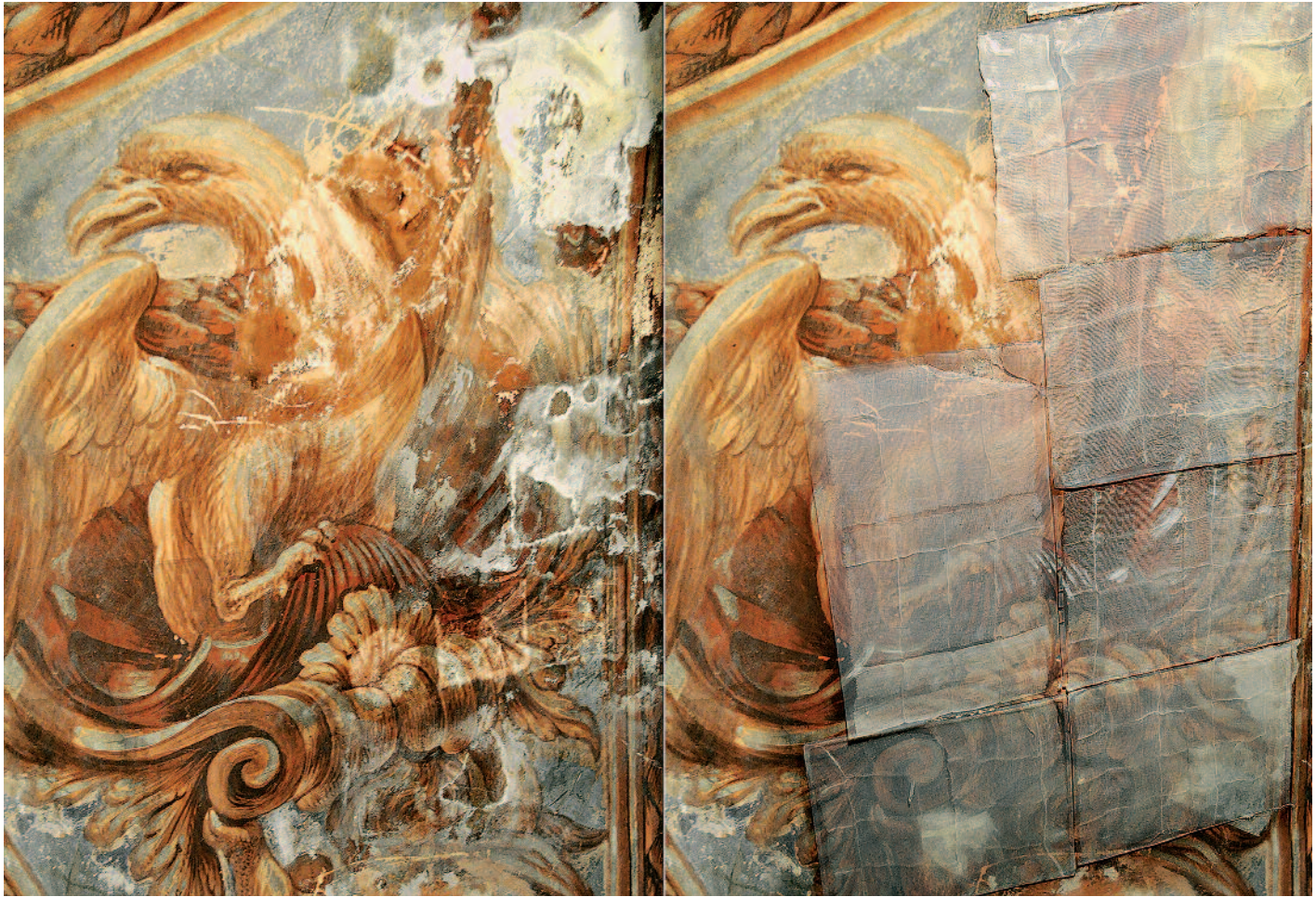
Salt efflorescence on a wall painting (left), example of salt reduction (right) on a wall painting by Antonio A. Palomino/ Guillo, Church of Santos Juanes, Valencia (Spain), 1698-1700; Photo: 2011, UPV
