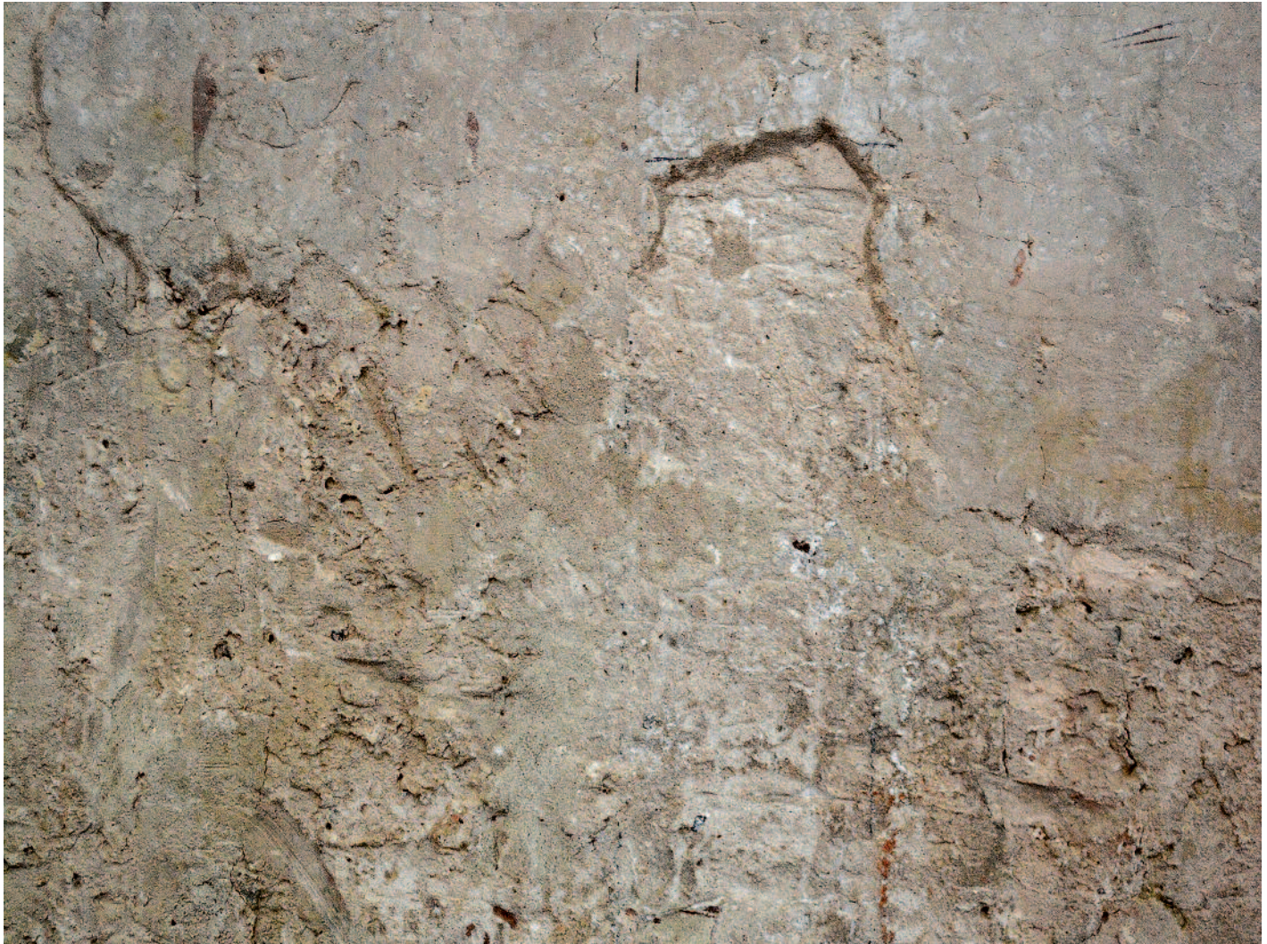
Coarse layer of arriccio (lower section) under intonaco, Chapel of St. Helen, Šenkovec (Croatia), late 14th century; Photo: 2014, HRZ (Katarina Gavrilica)
