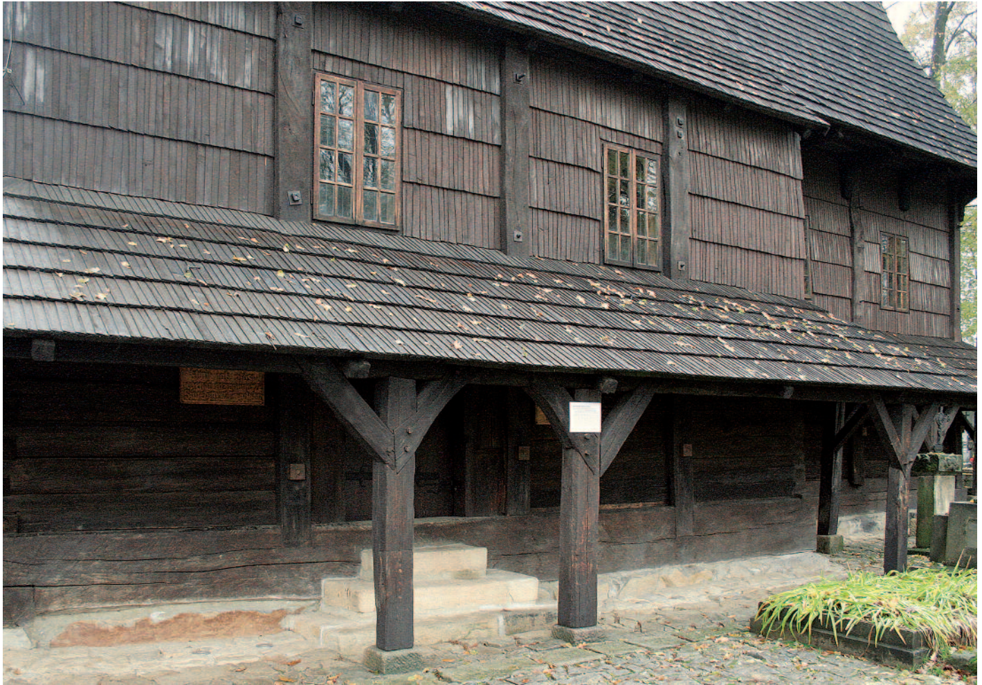
Façade and roofs with wooden shingles, Church of Saint Leonard, Lipnica Murowana (Poland), 15th century; Photo: 2008, UAD (Adrian Rauca)
