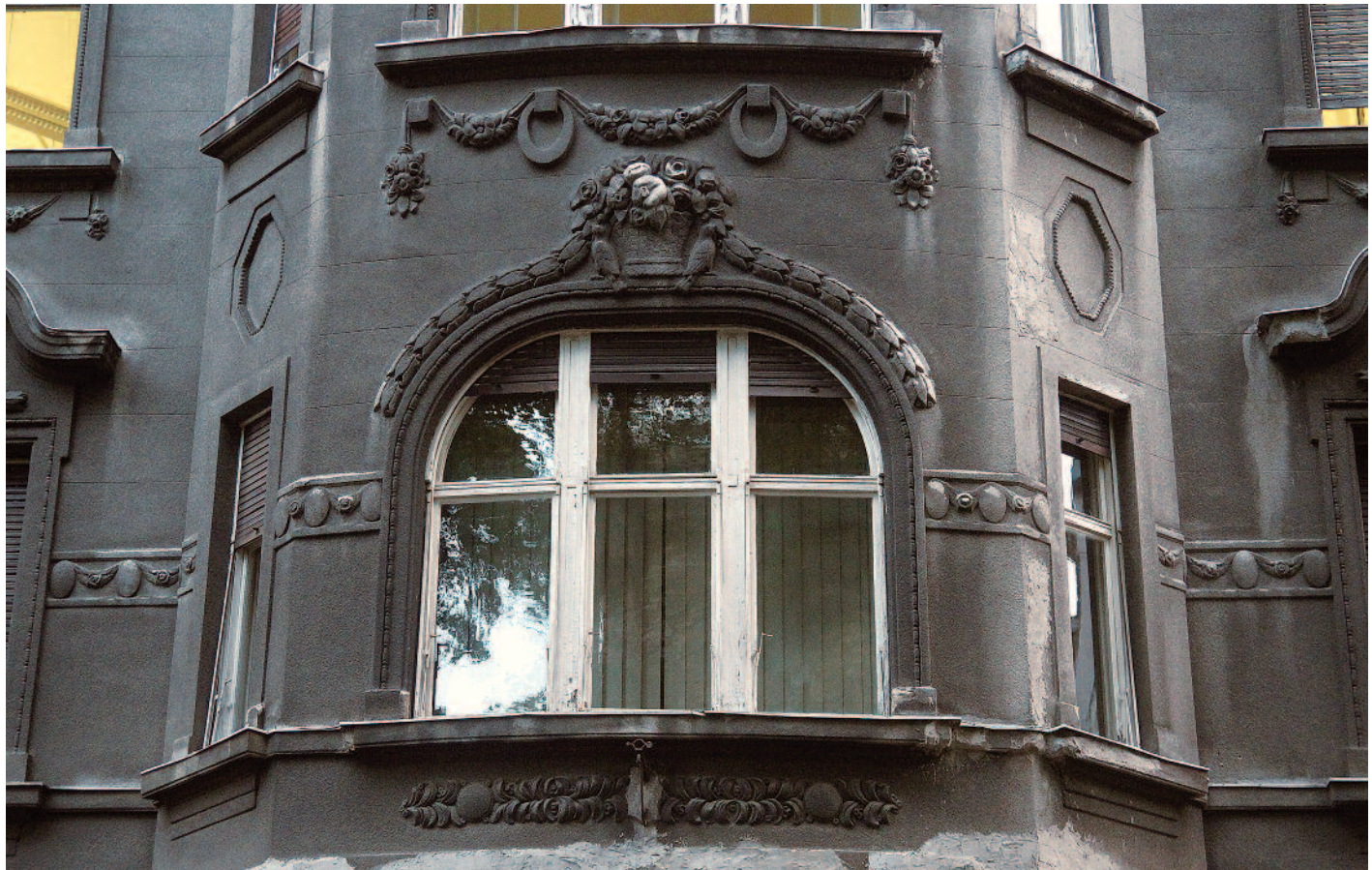
Darkened render on a façade, private building, Zagreb (Croatia), early 20th century; Photo: 2015, (Stefan Belishki)
