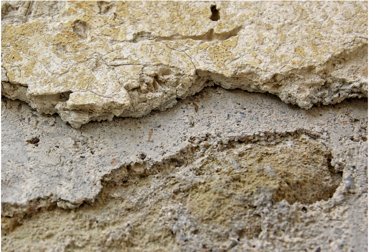
Levelling coat between masonry and finishing plaster (detail), Church of St. John Aliturgetos, Nessebar (Bulgaria), 13/14th century; Photo: 2014 (Stefan Belishki)
