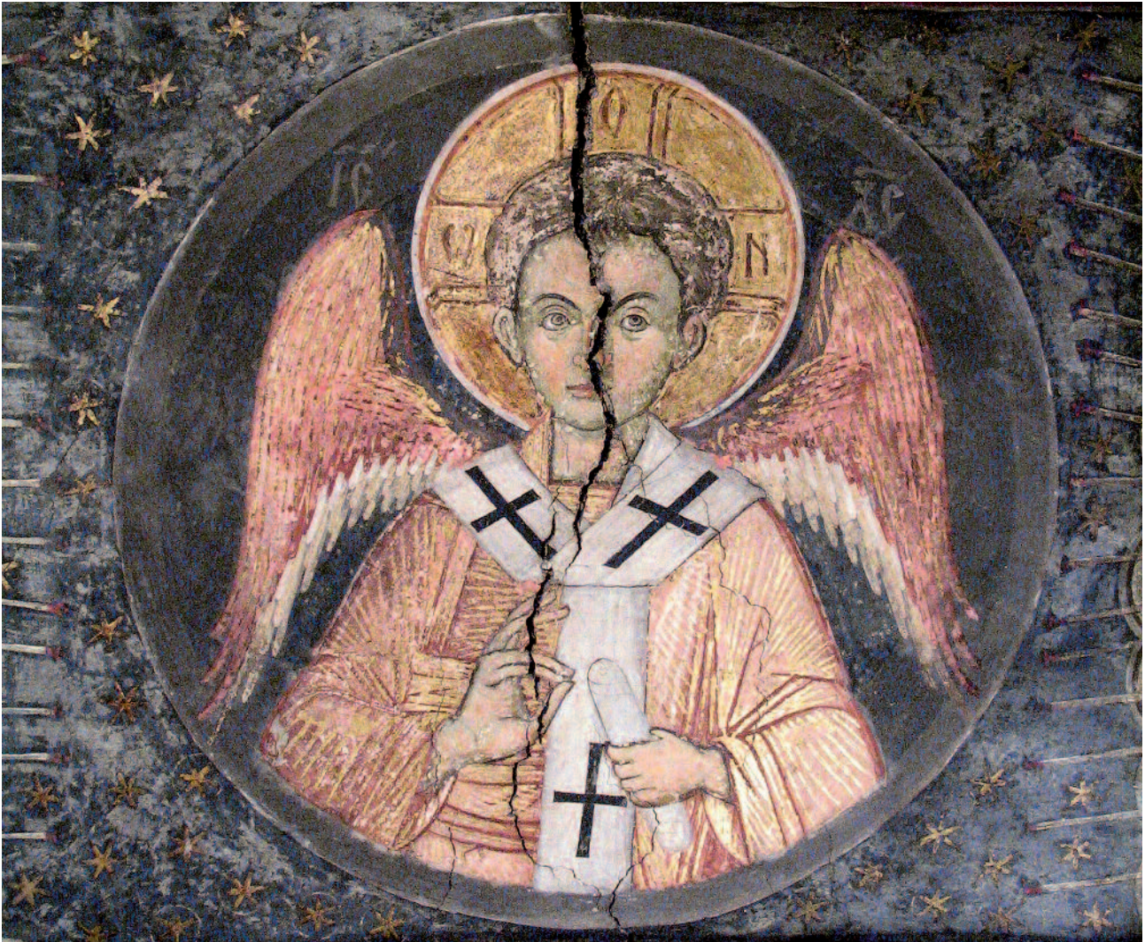
Crack in painted plaster, Sucevița Monastery (Romania), 1585; Photo: 2003, UAD (Adrian Rauca)
