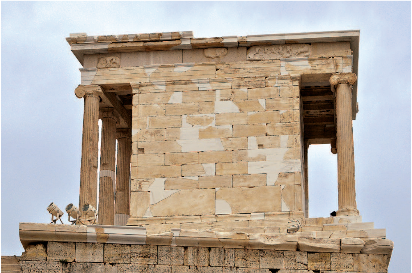
Marble inserts in the façade of the Erechtheion of the Acropolis, Athens (Greece), 421 and 406 BC; Photo: 2014, UPV (Pilar Bosch)
