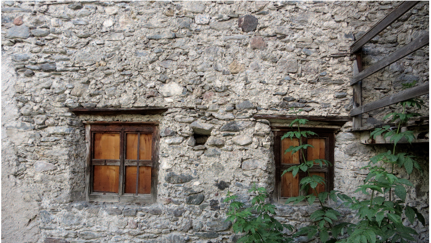
Typical rubble masonry, historic building, Santa Maria Val Müstair (Switzerland); Photo: 2015, HAWK (Angela Weyer)
