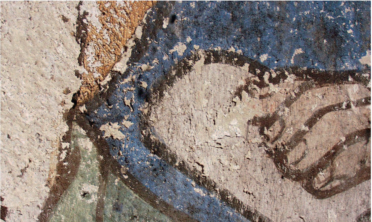
Monochrome ground under flaking paint layer, Church of St. Lorenz, Schöningen (Germany), 1904; Photo: 2001 (Barbara Hentschel)
