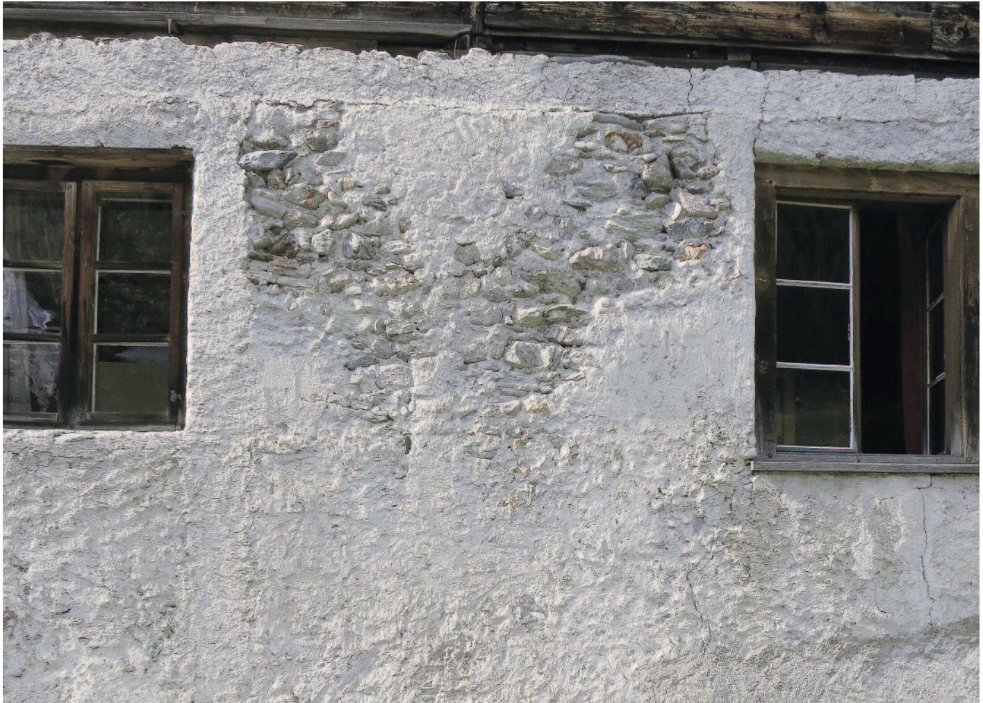
Rendered façade of historic building, Santa Maria Val Müstair (Switzerland); Photo: 2015, HAWK (Angela Weyer)
