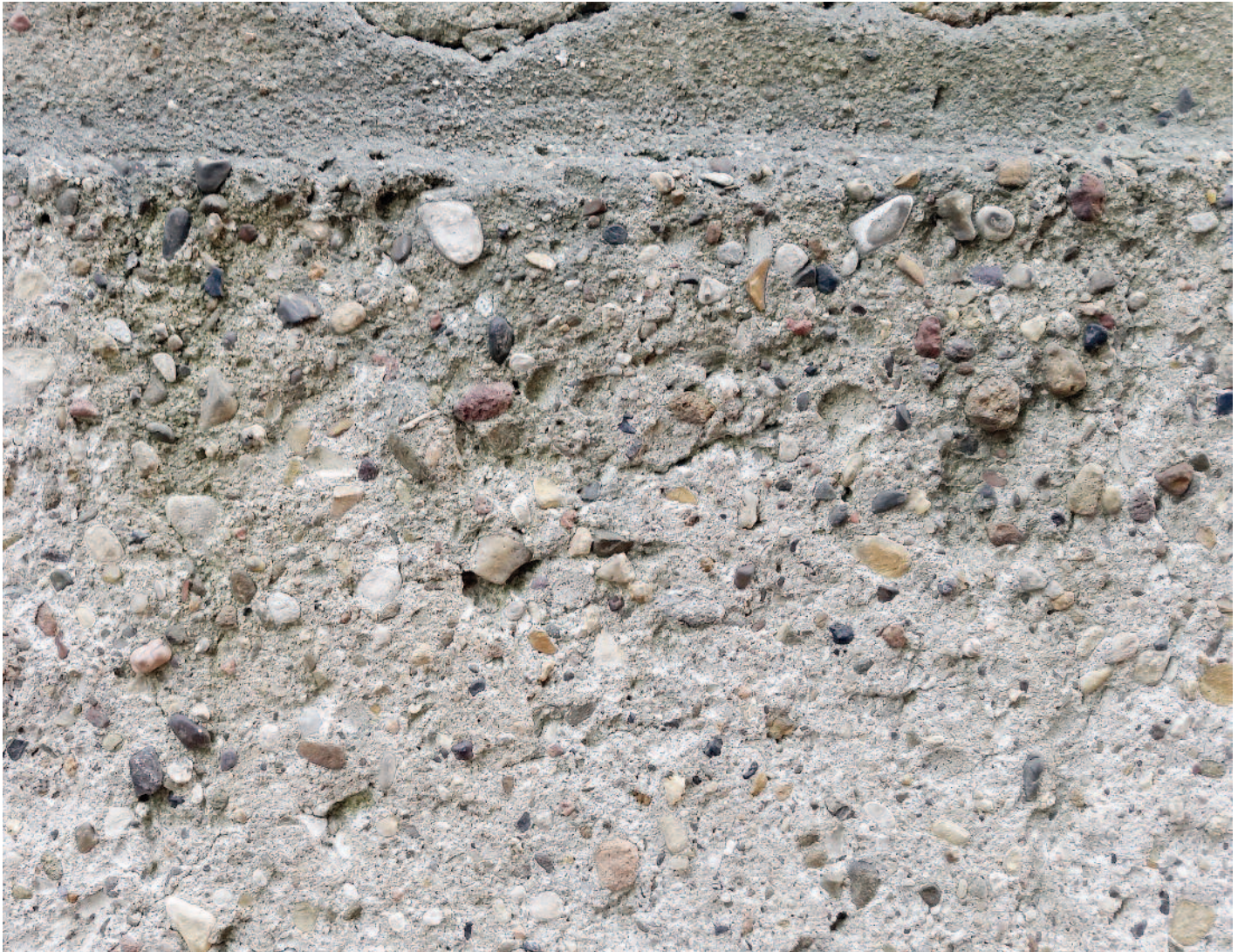
Detail of rough cast finish on an exterior wall, private building (detail), Hildesheim (Germany), mid-20th century; Photo: 2015, HAWK (Barbara Hentschel)
