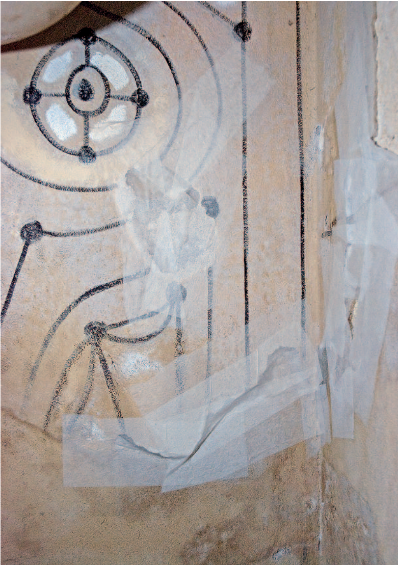
Facing applied to temporarily prevent scaling and delaminated areas from falling, chapel Saint Pierre, Villefranche sur mer (France), painted by Jean Cocteau, 1956/7; Photo: 2008, CICRP (Odile Guillon)
