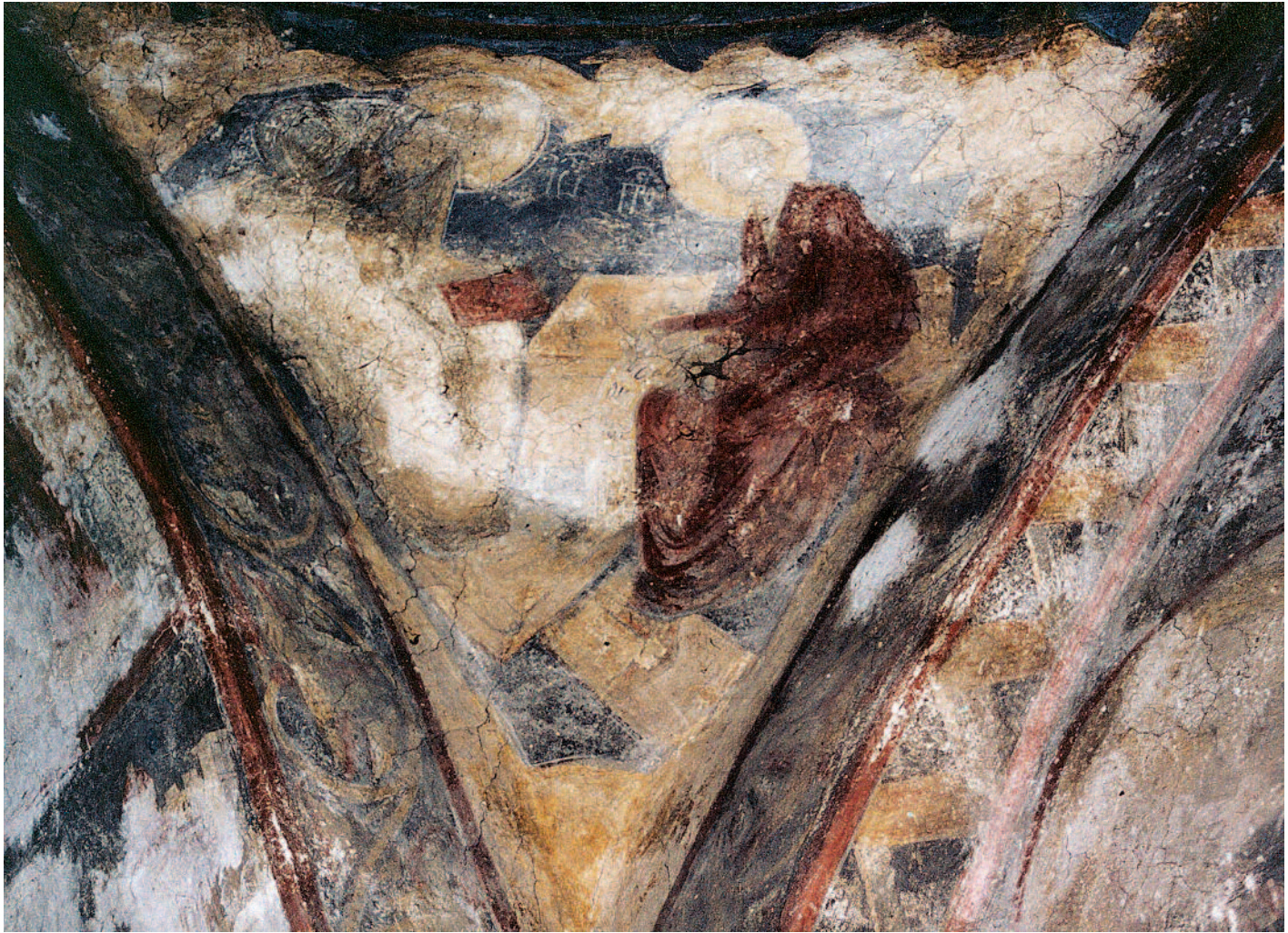
White haze on a wall painting, Moldovița Monastery (Romania), 1532; Photo: 1994, UAD (Theo-Sandu Mureșan)
